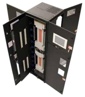
Sectionalized Layout in the eRPP-FSR Power Panel
